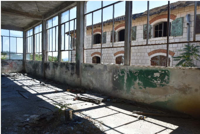
Figure 17: Shopfloor of the former Imota factory, Imotski
