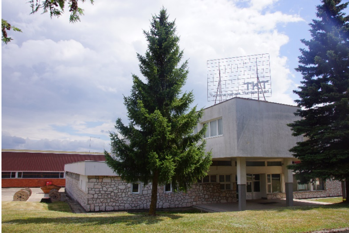
Figure 14: The TKT cable factory in Tomislavgrad
