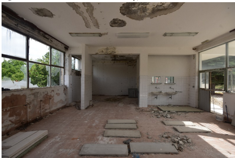
Figure 9: Inside the former Pionirka factory, Aržano
